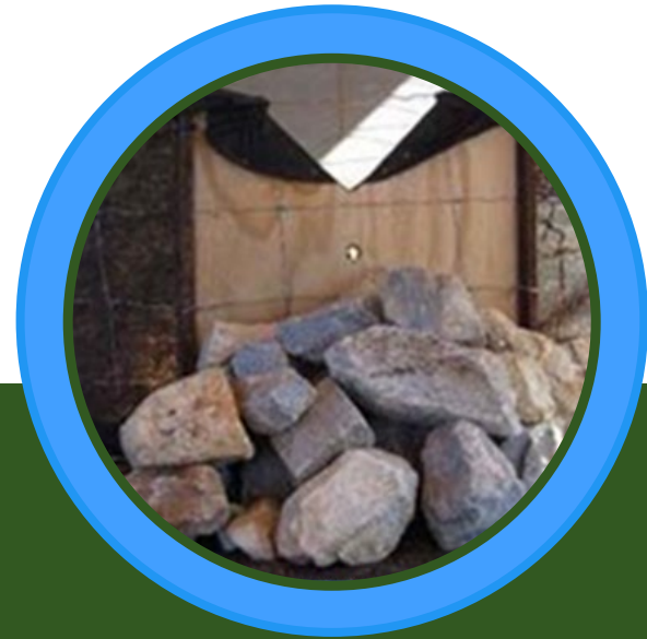
Weir & Dewatering Board
